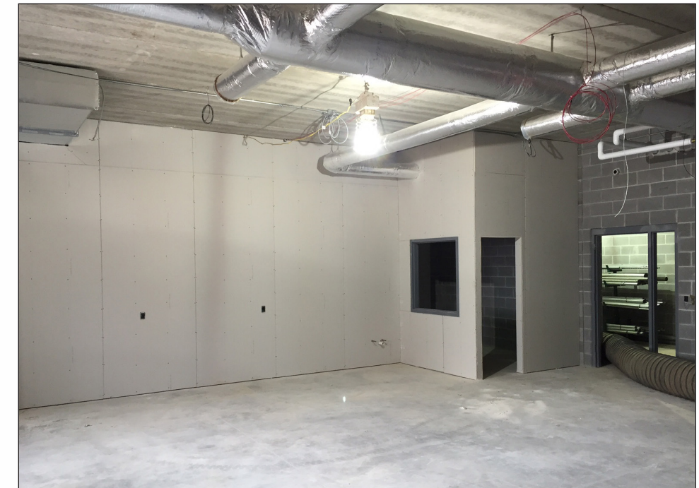
Classroom Ready for Paint
